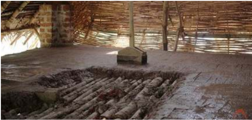
-Flat Mud Roof -Plinth protection using Lime
