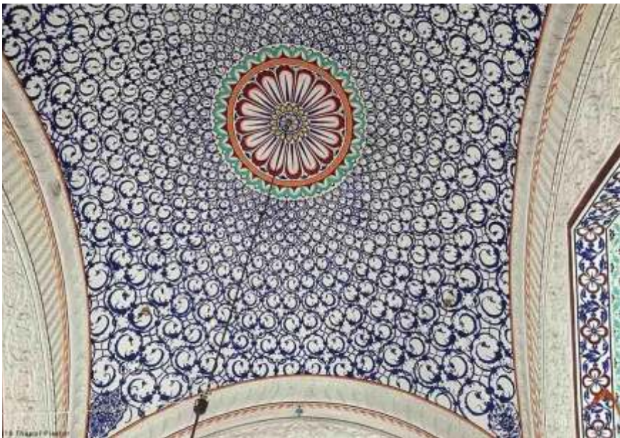
Revival of Thappi and Araish Plaster (Lime Plasters) -lime plaster thappi -lime plaster thappi araish
