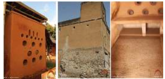
-18-feet high exposed Cob Wall protected with Thappi plaster -Research on Lime Stone Houses in Sardarshaher (Rajasthan) and Kankeyam (Tamil Nadu) -Lime Flooring
